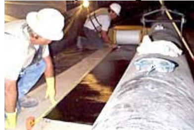
Photo: 5 (Patching with Repair Mortar)
