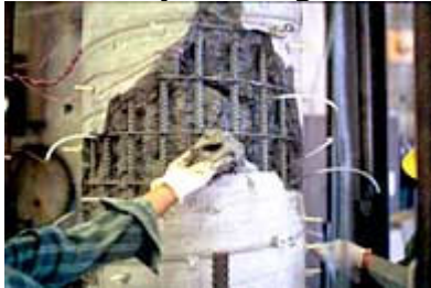
Photo: 4 (Patching with Repair Mortar)
